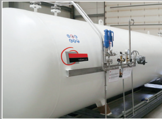
CO 2 high-pressure tank
