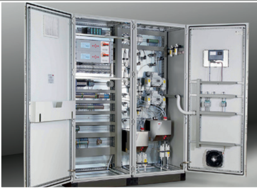
Gas analyser cabinet
