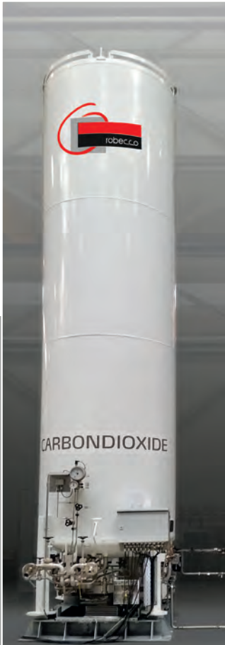
CO 2 low-pressure tank
